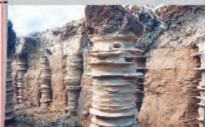
Jet-Grouting monofluido: acqua - cemento
