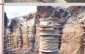
Jet-Grouting monofluido: acqua - cemento
